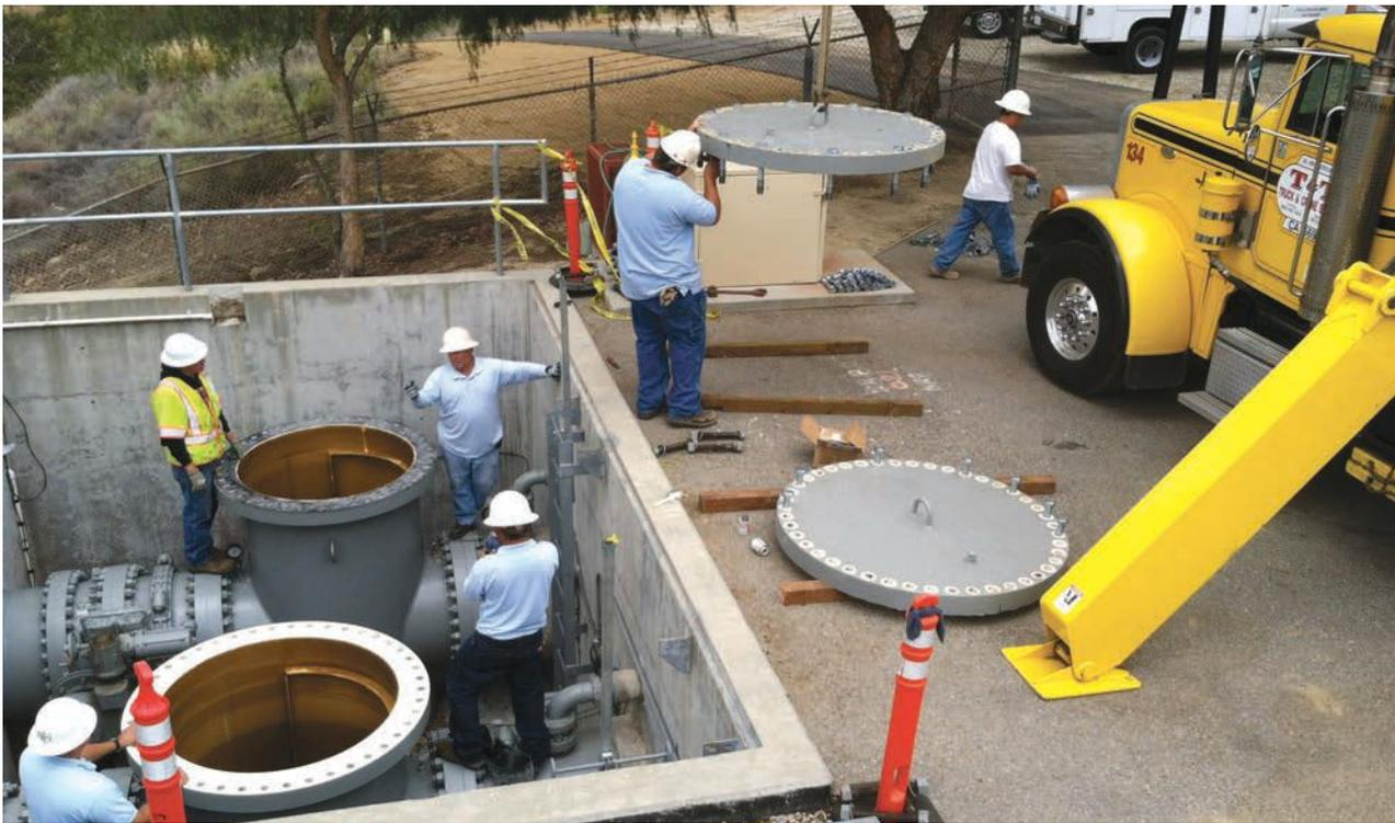
Above: Calleguas crews work to remove the protective inlet screens at the East Portal hydroelectric facility. Water supply conditions require the removal of these screens to keep the hydroelectric generator in service during periods of drought. Right: Archive images that show construction of the Calleguas water distribution system.
