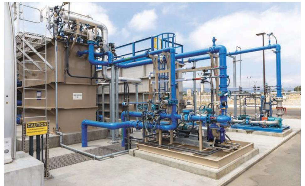
The new demonstration facility, above, uses a three-step process to purify treated wastewater into purified water. Data from this plant will be used to meet regulatory requirements for a full-scale facility that could eventually provide water to half a million homes. At top, the Los Angeles County Sanitation Districts Joint Water Pollution Control Plant in Carson.
