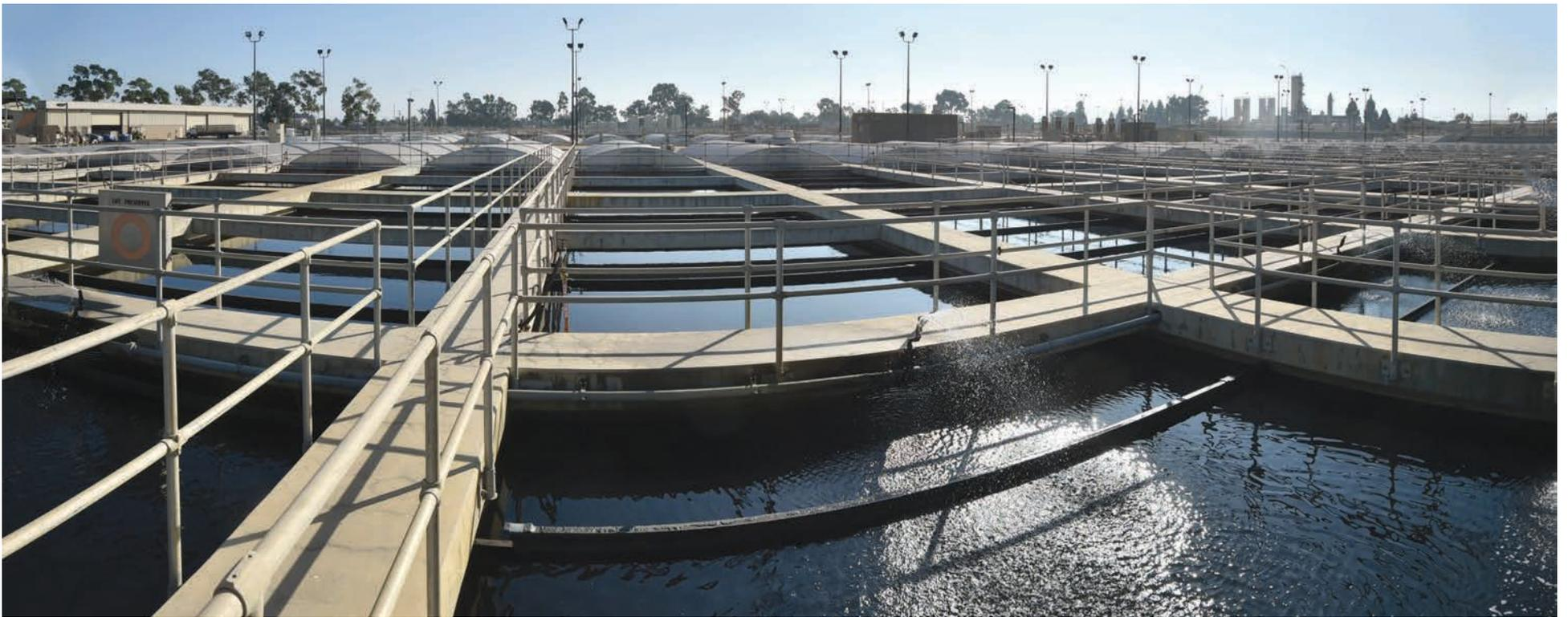
ocean. The demonstration facility purifies 500,000 gallons per day of the JWPCP's cleaned water using an innovative three-step process. First, membrane bioreactors remove ammonia along with other tiny particles. Next, molecules like salts are removed through reverse osmosis, which is the technology used for ocean water desalination. Finally, ultraviolet light and a powerful oxidant destroy any remaining pathogens and trace chemical compounds.
